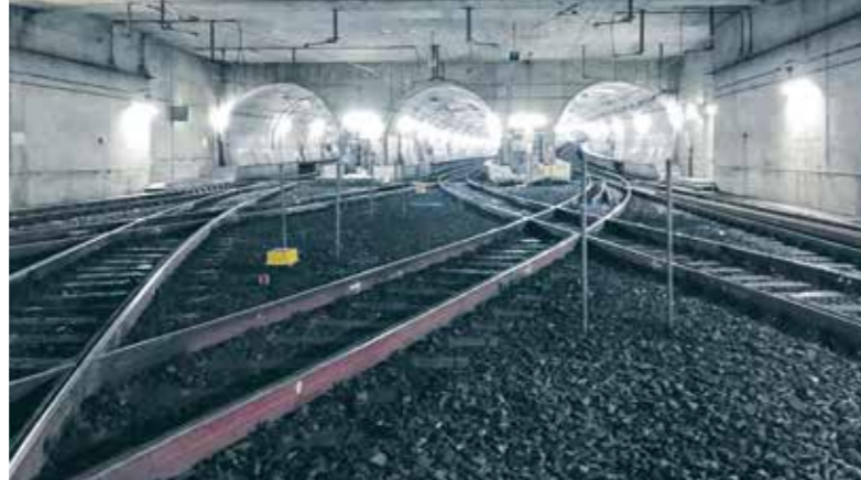
The reversing loop in the Frankfurt subway was also part of the construction work during the brief track closure in the summer.
