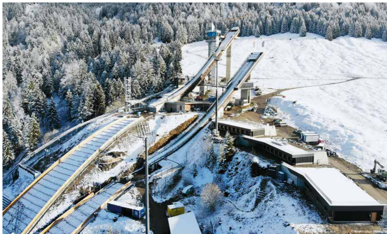
Restructuring work on the ski jump continues despite snow. The athletes' area is being rebuilt and the old ski jumps are being replaced with two smaller ones.
