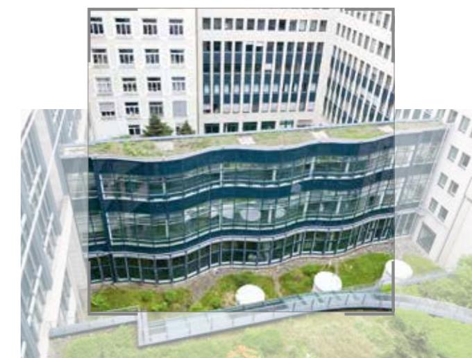
Drees & Sommer developed future scenarios for the Norderstrasse 101 building in Hamburg, the largest property in the portfolio by far.
