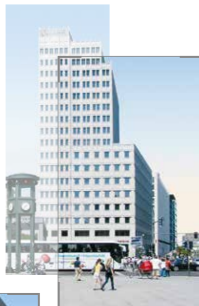
Unmistakably Berlin: The real estate experts carried out a thorough inspection of the high-rise building Potsdamer Platz 5.
