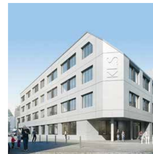
One of the buildings at the Palmstrasse school campus in Cologne’s city center has already been rebuilt.
