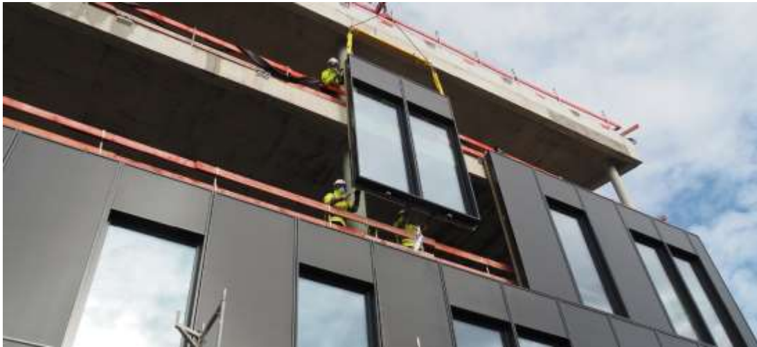
The façade can also be installed in buildings with a height of more than 20 meters. ©Drees & Sommer SE
