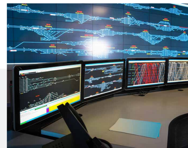
Digital train control system
