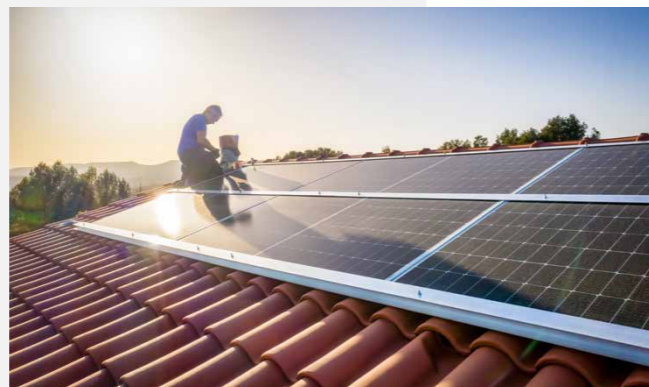
Photovoltaics on buildings
