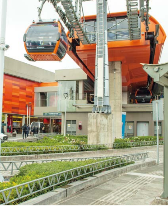
Examples of different station constructions (La Paz, Koblenz and London)
