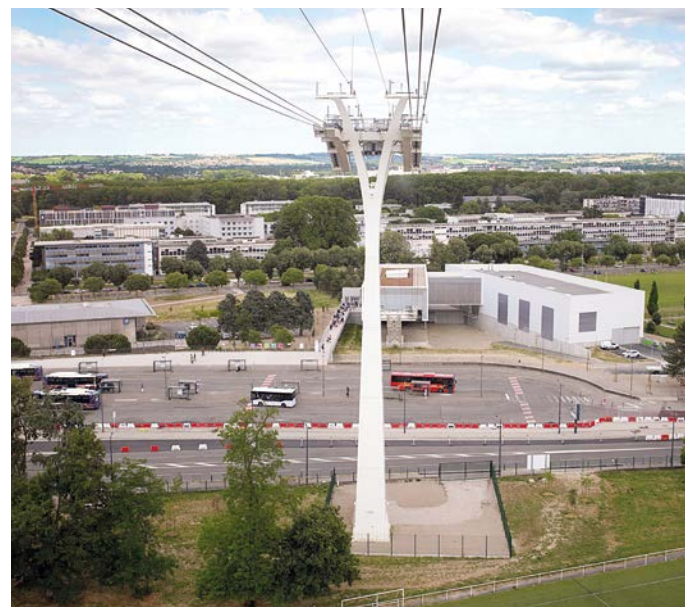
Examples of different pylon constructions (Brest, Toulouse)
