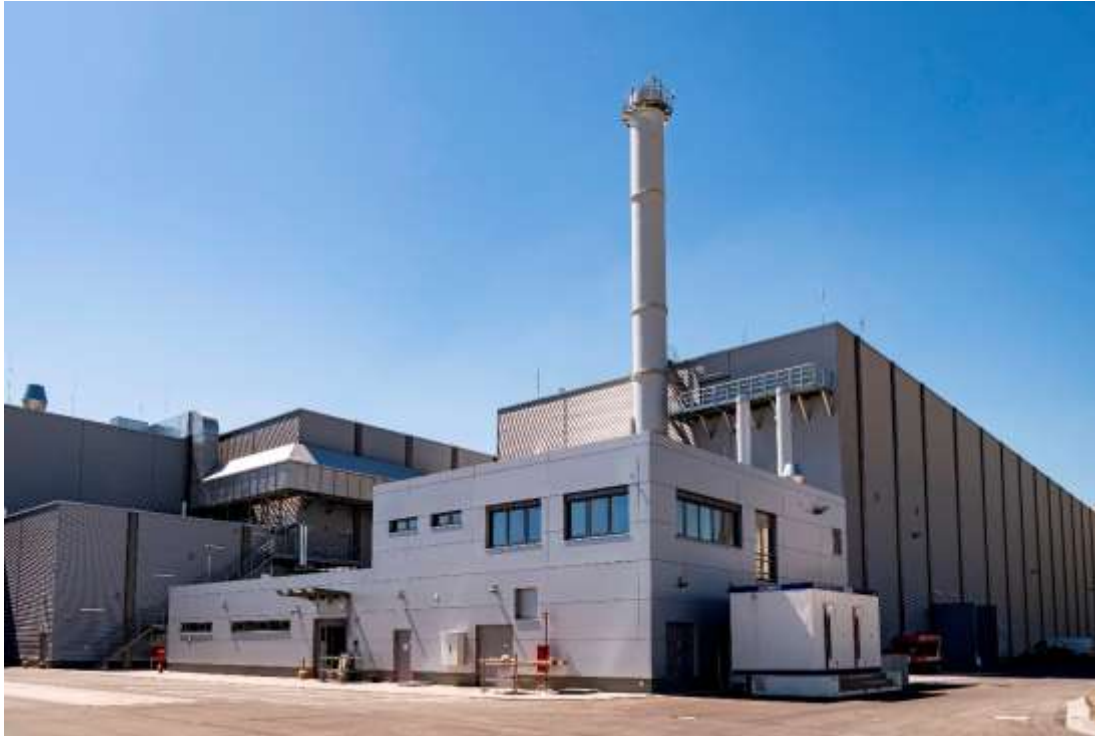
The Philippsburg residual material processing center received commissioning approval back in December 2020. Photo: EnBW Kernkraft GmbH
